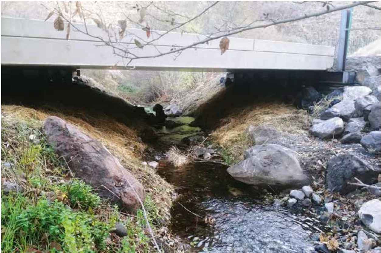
Downstream view of Bridge Replacement Project with steelhead passage barrier removed.
