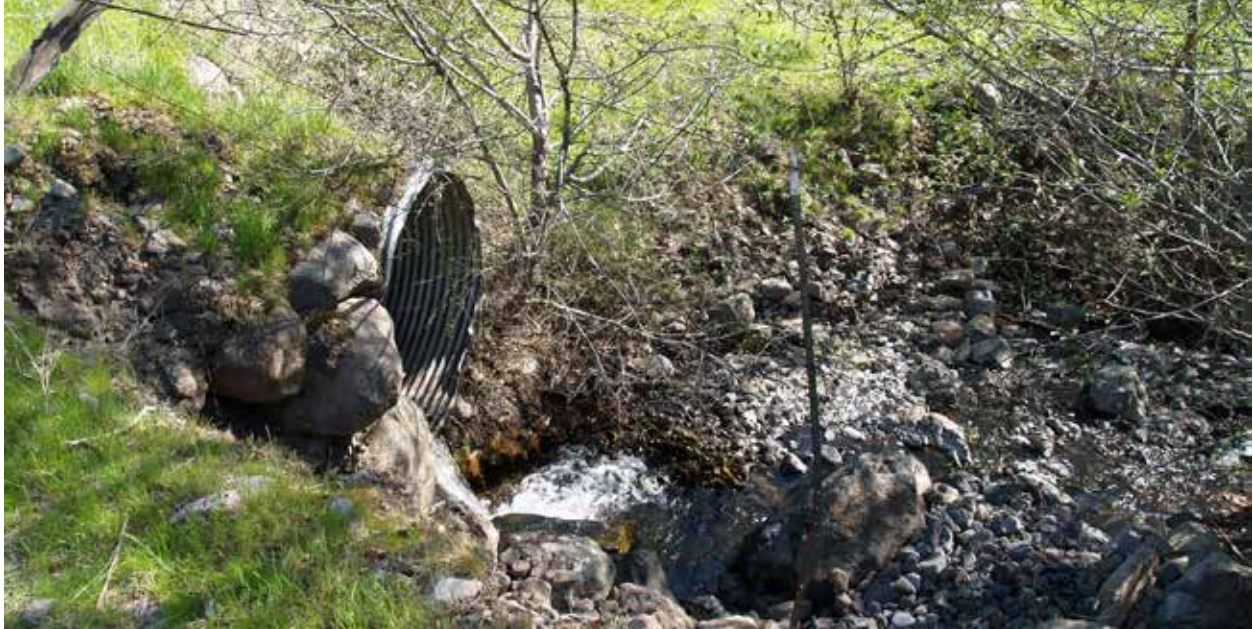
Outlet of Perched Culvert before Bridge Installation
