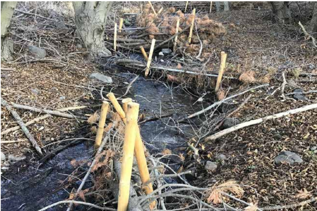
Example of 5 different PALS structures above the bridge. Bridge would be in bottom left of above photo
