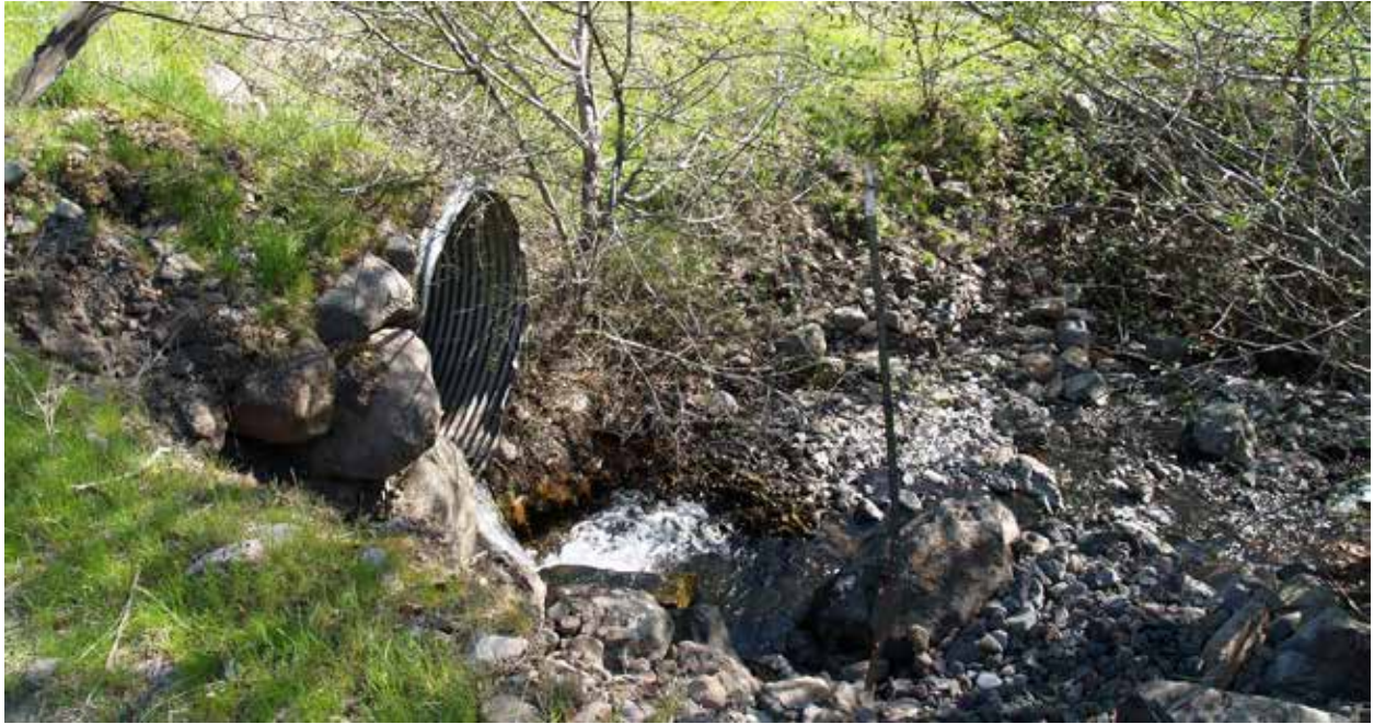
Outlet of Perched Culvert before Bridge Installation
