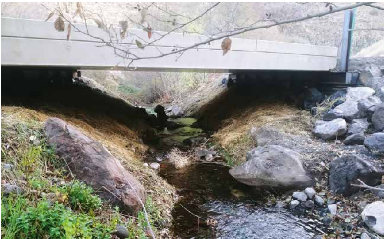
Downstream view of Bridge Replacement Project with steelhead passage barrier removed.
